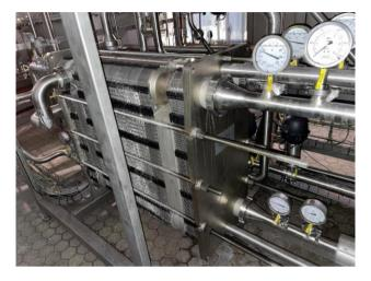
In the 3<sup>rd</sup> section, forming gas was introduced on the glycol side T4 and T3. Compressed air was applied to the beer side. No forming gas was detected in the compressed air circuit. A 'sniffer' (sensor) was used all around this section. No external leaks were found.
