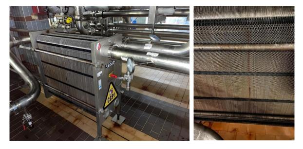
There are 279 plates in the cold block cooler. The actual installation size (after tightening) is 934 - 935mm.
